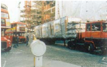
Delivery to the project site.
