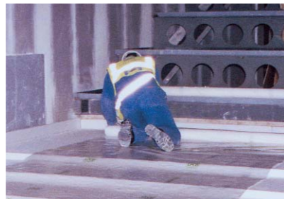
IAC designed and installed five studios with Acoustic Panel System Floating Floors for Radio City's new station headquarters at the top of the 137m high St. John's Beacon in Liverpool city centre.
