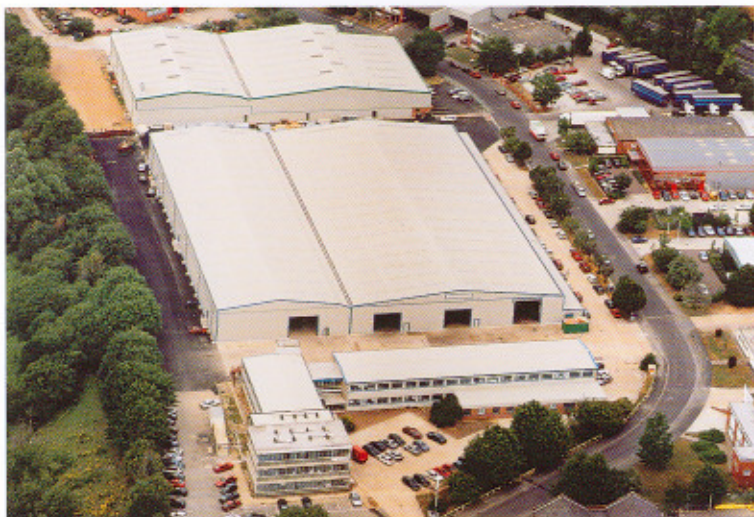
Pictures above and below show IAC's production plant at its European Headquarters in Winchester, UK
