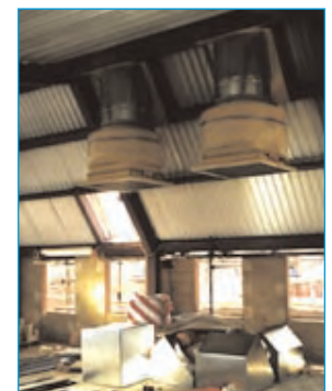
Figure 7.9.2: The roof terminals, viewed from inside during construction
