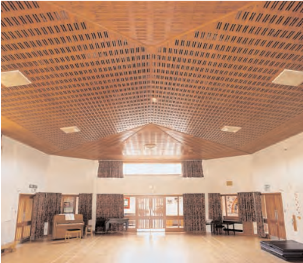
Figure 7.1.3: The hall ceiling after acoustic treatment
