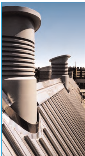
Figure 7.9.4: Three of the roof terminals, during construction
